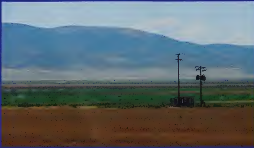
A shed houses a well that provides water for agricultural irrigation. Other irrigation wells have been converted to municipal supply as the population of the valley increases. Lake Mountains in the background.
